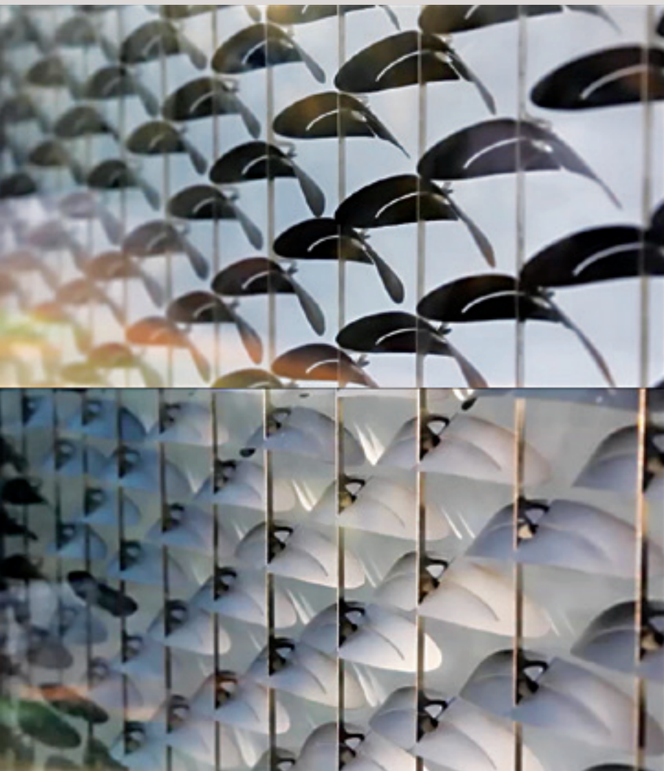
InVert Windows , in progress Thermobimetal, stainless steel, insulated glass Dimensions variable Self-shading double-glazed window system
