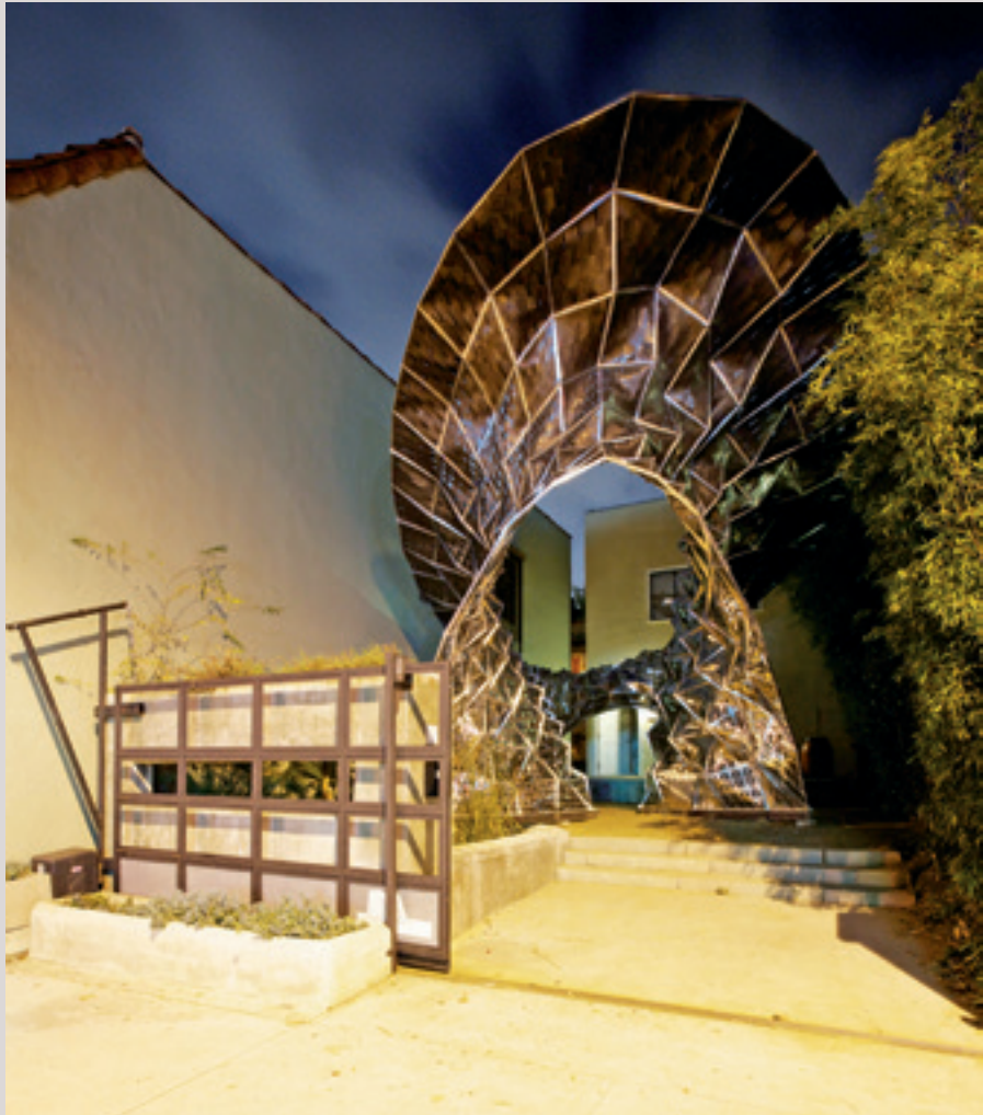
Bloom , 2011 Thermobimetal, aluminum, steel 21 x 20 x 40 feet A lightweight monocoque structure sheathed with a sun-shading, self-ventilating surface that responds to the moving sun Photo: Brandon Shigeta
